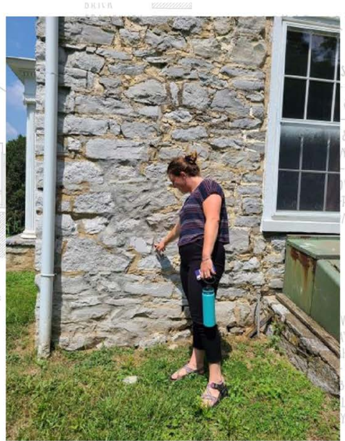
Lydia pointing out Portland cement used on Fort Bowman's side elevation.
