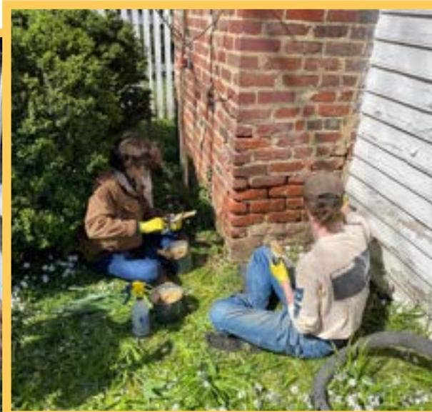
After removing harmful Portland cement by hand, students apply fresh lime mortar to sections of the Mary Washington House foundation
