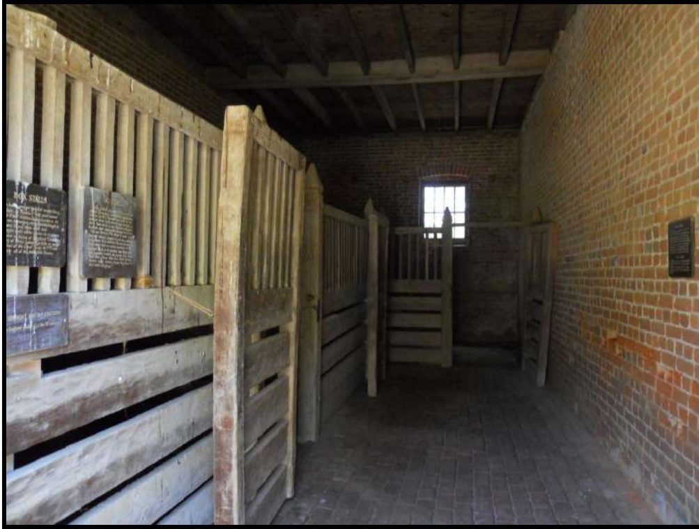
Figure 6 depicts the box stalls at Stratford Hall. These stalls were used for horses that had to be kept inside for an extended period of time. Note the lack of fenestration in the exterior wall on the right.
