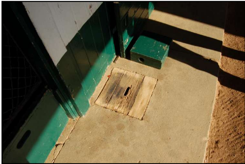
Figure 46 shows a recess in the floor for soaking or poulticing hooves.
