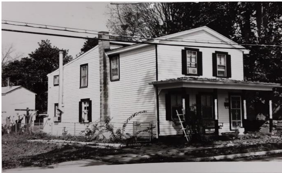
The former Thornton Residence at 519 Hanover Street in 1985. Photo by Mary Beth Gatzka (Class of 1987).
