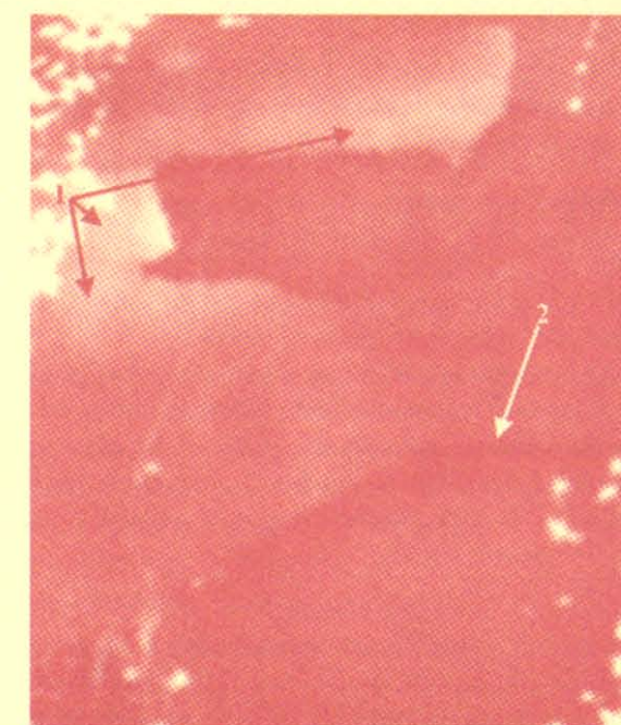
Picture of the UMW amphitheatre taken by Liz Fedowitz, Erin Glennon, and Katie Hummelt. The number one arrows point to bright spots that show delamination occurring in the cement. The number two arrow shows the outline of the steps that were attached at one point but since removed.
