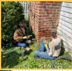
After removing harmful Portland cement by hand, students apply fresh lime mortar to sections of the Mary Washington House foundation
